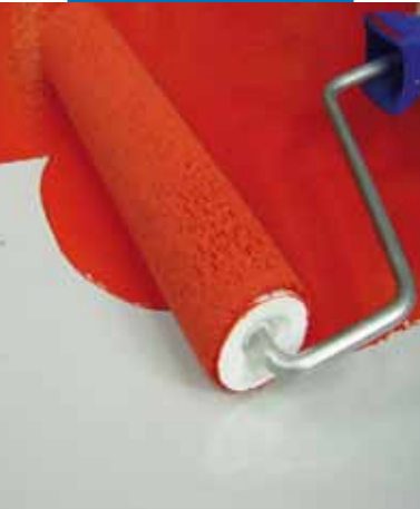
Application of Mapecoat PU 15 with a roller
