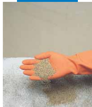
Spreading dry sand on fresh Mapecoat I 24
