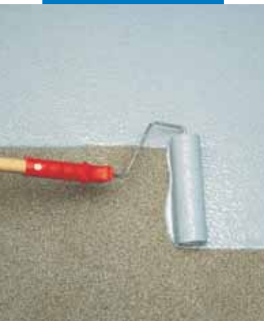
Applying Mapecoat I 24 with roller
